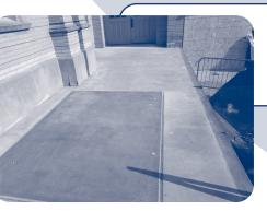
Water Treatment Plant Loading Dock Rebuilt the loading dock to replace the original 1920s dock. Added an access hatch for future boiler replacement
