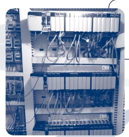
New Programmable Logic Controllers (PLCs) PLCs in the water plant were upgraded to meet current standards for computerized equipment control
