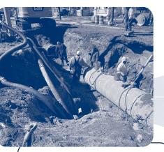
Maintenance and Service Crew repaired a blow-out on a 36-inch transmission main
