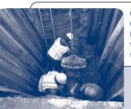
**Gratiot Pump Station** Crew replaced an inoperable valve to improve station function
